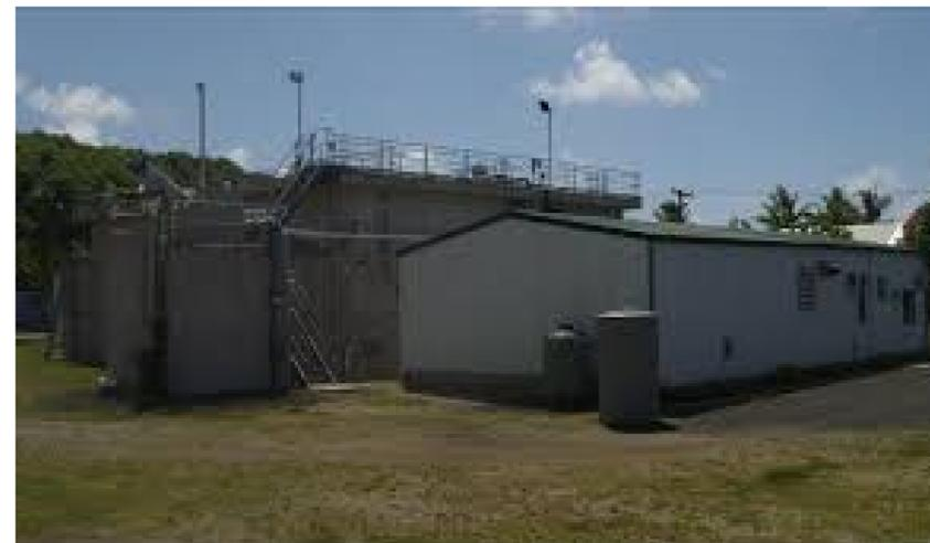
Installed in 2009, this system manages wastewater collected from Samoa's central business district area. It uses a wastewater treatment plant (tertiary treatment), and the plant's capacity is about the same as would be needed to service Muri. This treatment plant replaces septic tanks (which are still the main treatment system around the island) and was installed in response to poor quality of Vaiusu Bay.
