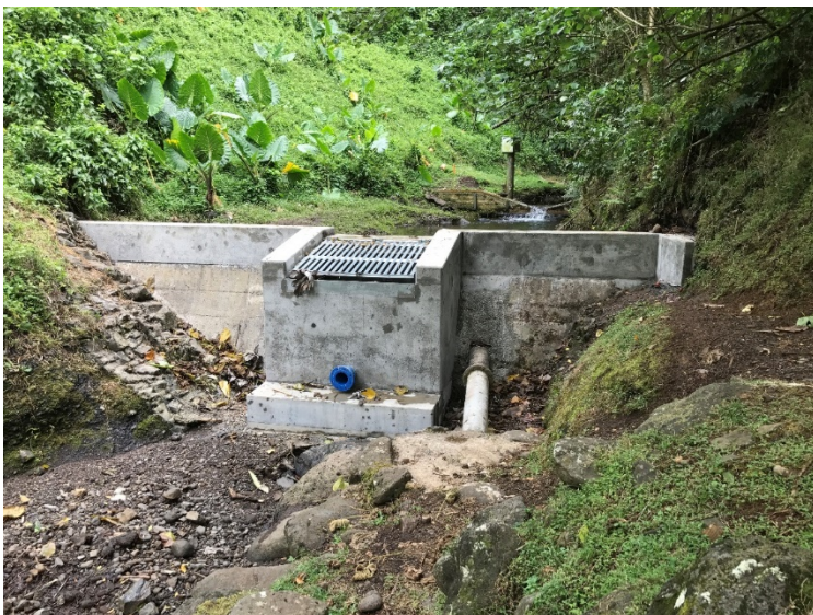
The intake structure at Matavera
