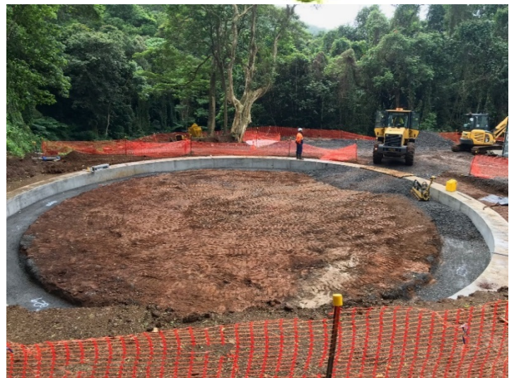
Completed earthworks and concrete ring beams for the new storage tank
